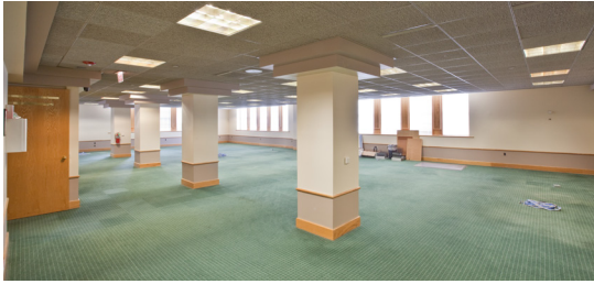
Part of the library space before renovations. Simon Hurst Photography
